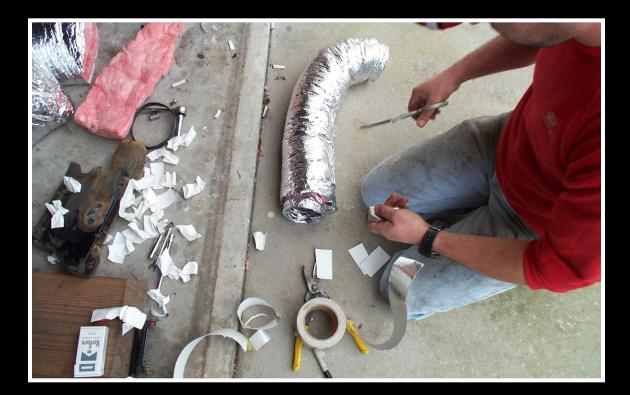
Here we have Carl and mylar tape again. Hes cutting off pieces to secure the insulation and outer layer to the inner. (Sorry ladies, but this man is taken!)
