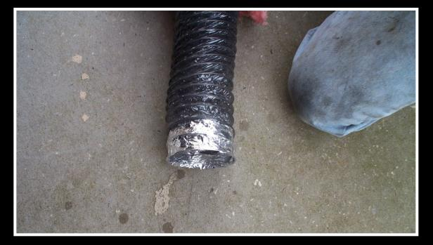
First, roll or push the insulation back to reveal the ducting itself. The end should appear fairly fragile, so we reinforced it with mylar duct tape.s Use whatever you have to make the end sturdy. As the inlet, you want it to be able to handle whatever speed air is thrown up through your intake.
