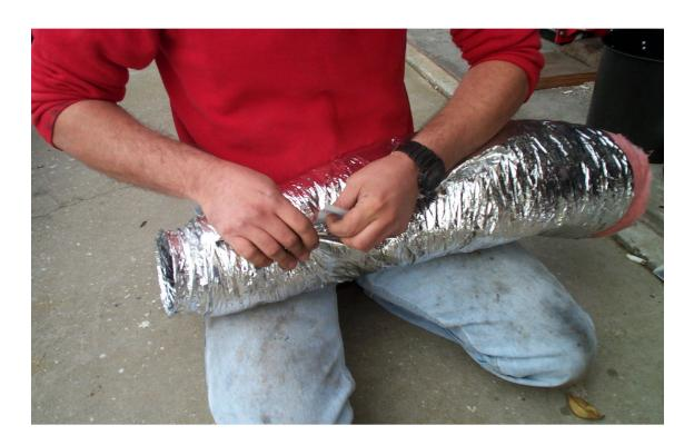
Here were using the "pinch and roll" method of controlling the thickness of the ducting. Why let all that insulation be puffy when you can make it lean. Simply pinch the insulation down to the duct underneath, then fold, and tape down (again with the mylar duct tape). You'll be repeating this along the entire length.
