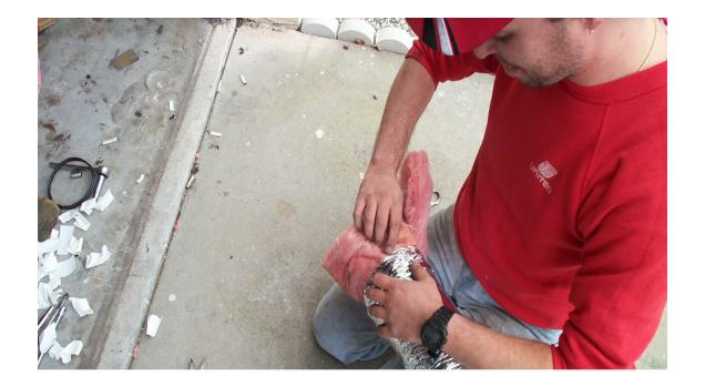
When you've gotten to the end, you'll doubtlessly have "leftover" insulation at the end. Simply cut and remove this extraneous material, and consider yourself almost finished.
