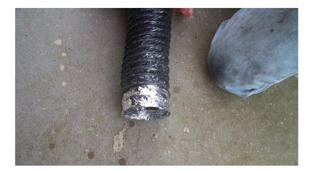
First, roll or push the insulation back to reveal the ducting itself. The end should appear fairly fragile, so we reinforced it with mylar duct tape.s Use whatever you have to make the end sturdy. As the inlet, you want it to be able to handle whatever speed air is thrown up through your intake.
